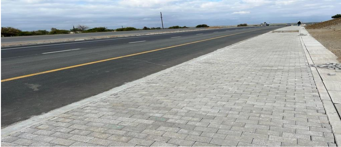
Beitbridge Road Dualization (urban section with a foot path)
